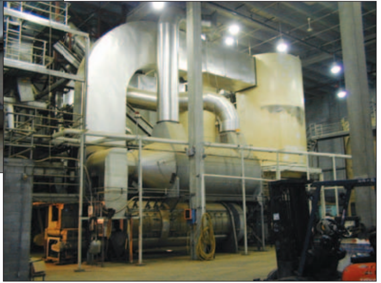
A high-capacity sludge drying plant in the USA. In this configuration, the hot air generator is positioned above the AST Dryer.
