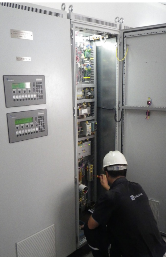
Coromax control cabinet
