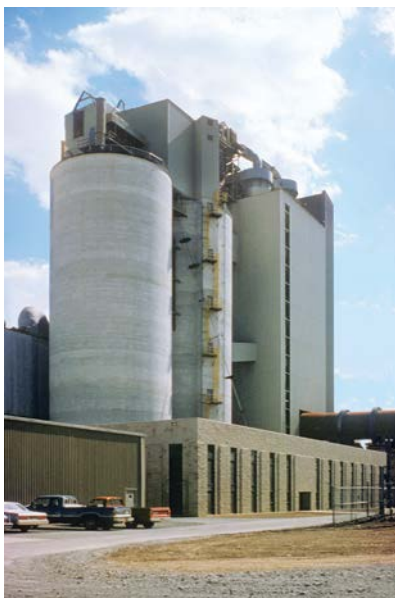
Airmerge™ blenders at a USA cement plant
